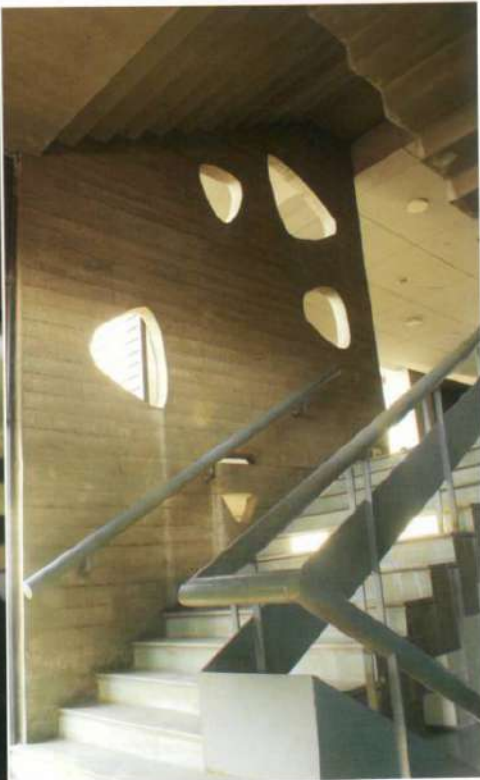
“ The stair façade punctures in exposed R.C.C, inspired by legend Le Corbusier, The punctures allows the southern air to flow in building with symphonic force. ”
