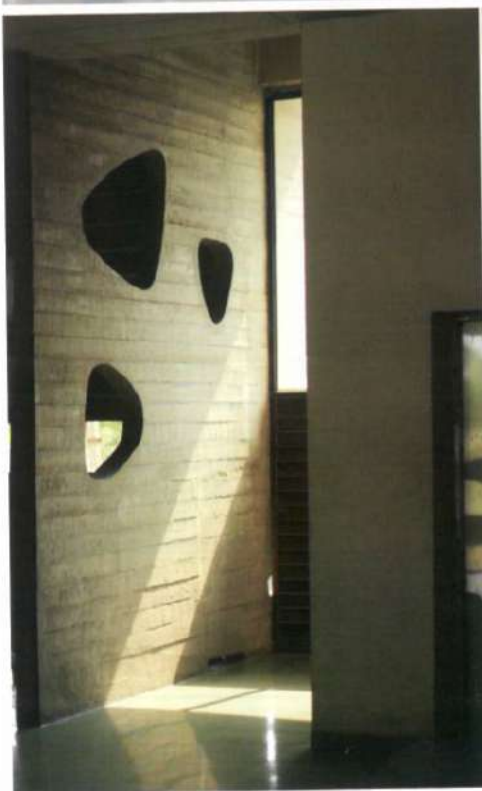
“ The stair façade punctures in exposed R.C.C, inspired by legend Le Corbusier, The punctures allows the southern air to flow in building with symphonic force. ”
